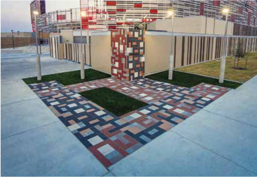
The "Cougar Pride" walkway consists of 19 precast concrete panels, comprising four vertical and 15 horizontal panels created with an artistic mosaic of "U" and "H" figures in different color combinations. Photo: Jim Isemann
