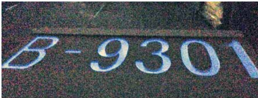
This architectural precast concrete panel had glow-in-the-dark aggregates post-applied to the interior of the numerals cast into the panel to serve as the building's address. Photo: Gate Precast
